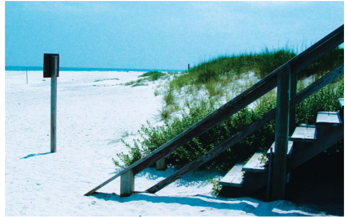
Photo 19: The steps were intentionally buried at the time of construction.
